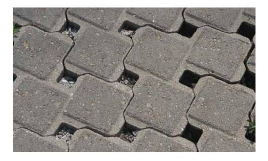
Porous surfaces can be thought of as a rigid, load bearing area with an internal structure not unlike open cell foam. When water comes in contact with the upper surface, it flows immediately through the surface to the engineered volume under it.
